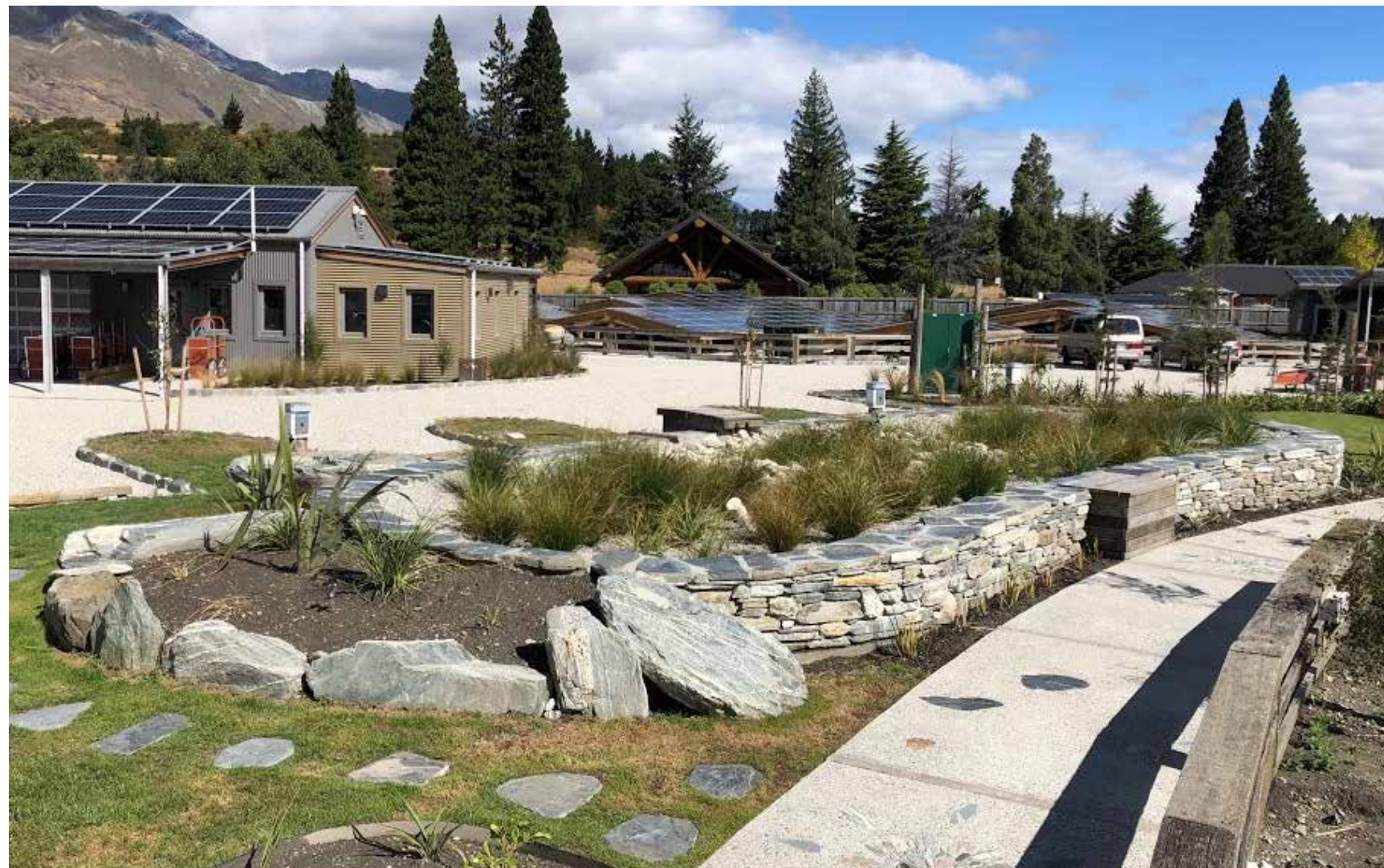
Above: The 'Solar Farm' that powers many of the facilities in the campground. Top: A typical cabin at Camp Glenorchy, complete with a porch and native vegetation. Right: The largest bioswale on site, collecting and treating grey water from campers.
