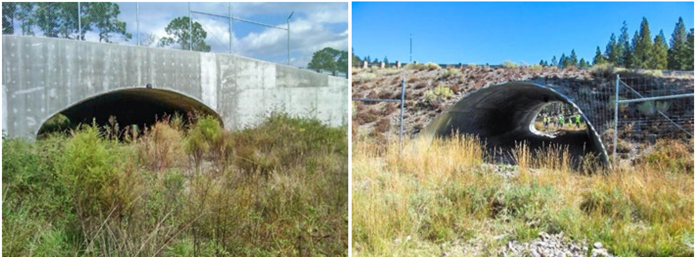
Figure 8-5 Examples of large arch culverts in upland communities (left, Immokalee Road in Collier County; right, California). The Immokalee Road crossing includes angled wing walls.
