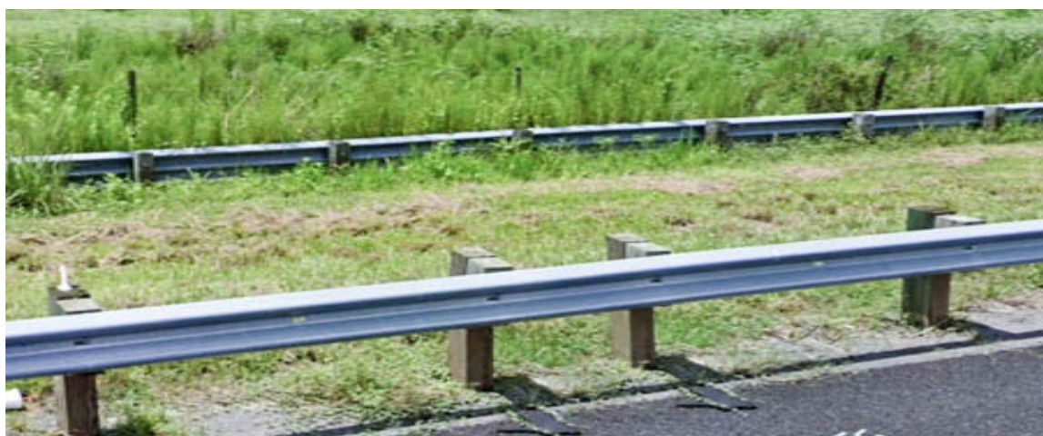
Figure 3-30 Installation of thrie-beam guardrail (in the background) used as a barrier to prevent trespass by small mammals and herpetofauna in Paynes Prairie State Preserve.
