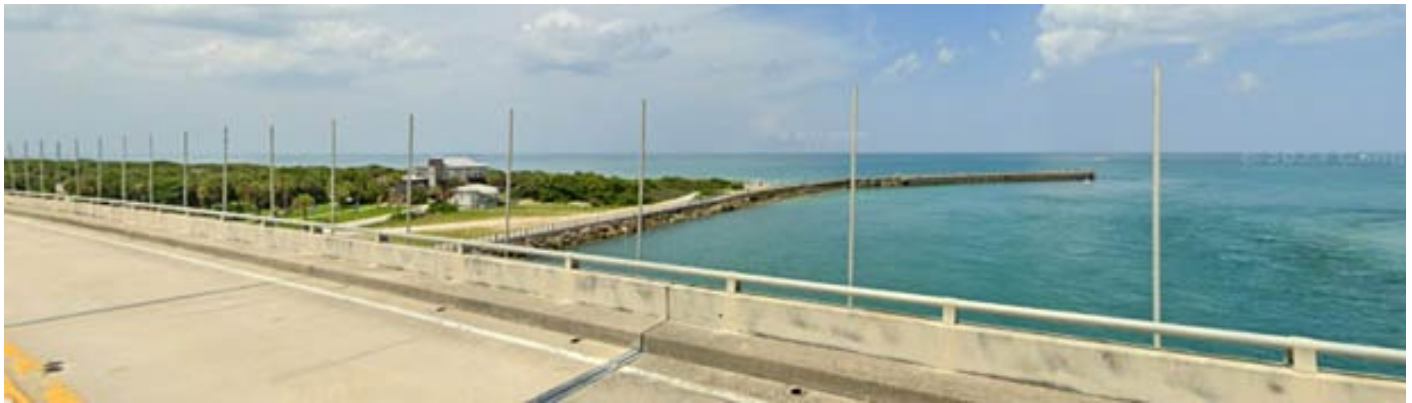
Figure 3-47 Metal poles installed on the A1A bridge over Sebastian Inlet. They encourage flight paths above oncoming traffic (although Royal Terns were the subject of this measure, it has positively influenced other species too).
