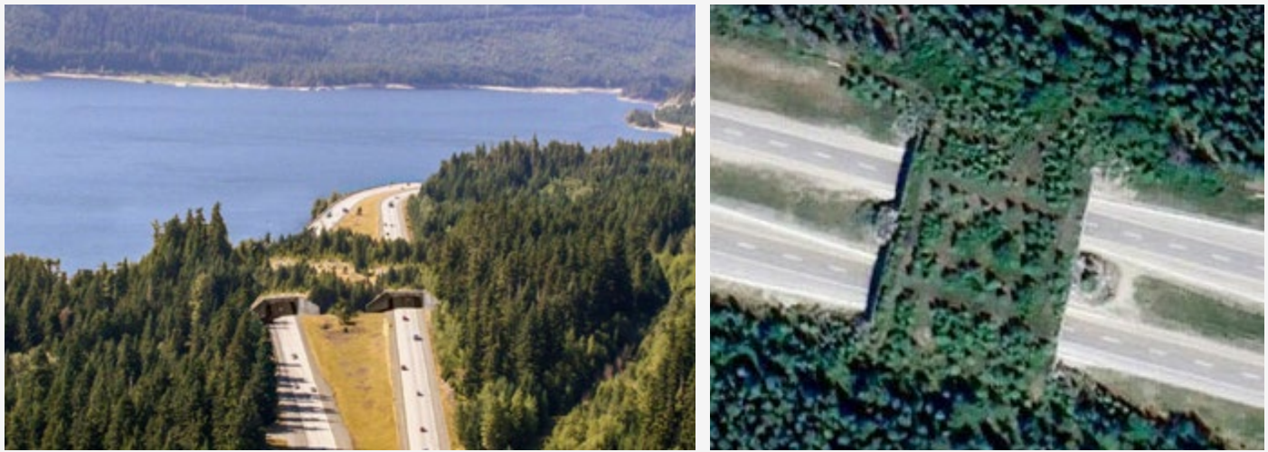
Figure 8-2 Additional examples of wildlife overpasses (in Washington [left] and Europe [right]); note the use of landscaping to provide cover, clear zones in the center on the left and more dense plantings across the structure on the right. Also see figs. 3-1, 3-2 and 3-5 to 3-10 . Photo source: WSDOT , left.
