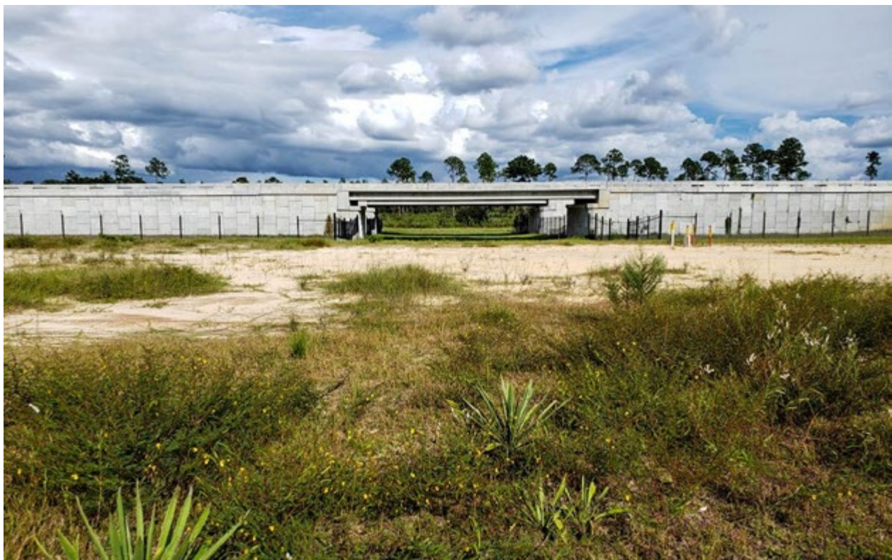
Figure 3-4 An example of wildlife fencing. Designed to direct animals toward crossings and away from traffic lanes.
