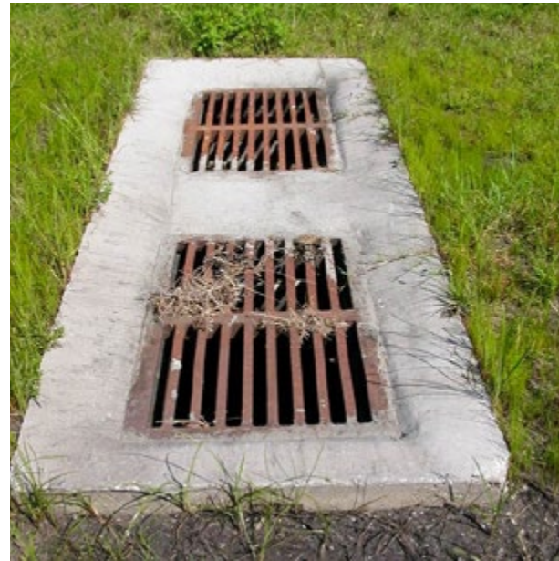
Figure 3-20 An example of a steel grate; installed to allow light penetration in the center of the culvert tunnel.
