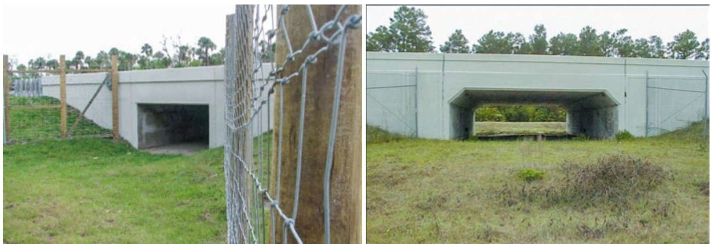
Figure 8-4 Small (<5 ft) and large (> 5 ft) box culverts in upland communities (left, SR 60 in Indian River County; right, SR 46 in Lake County). Also see fig. 3-19d .
