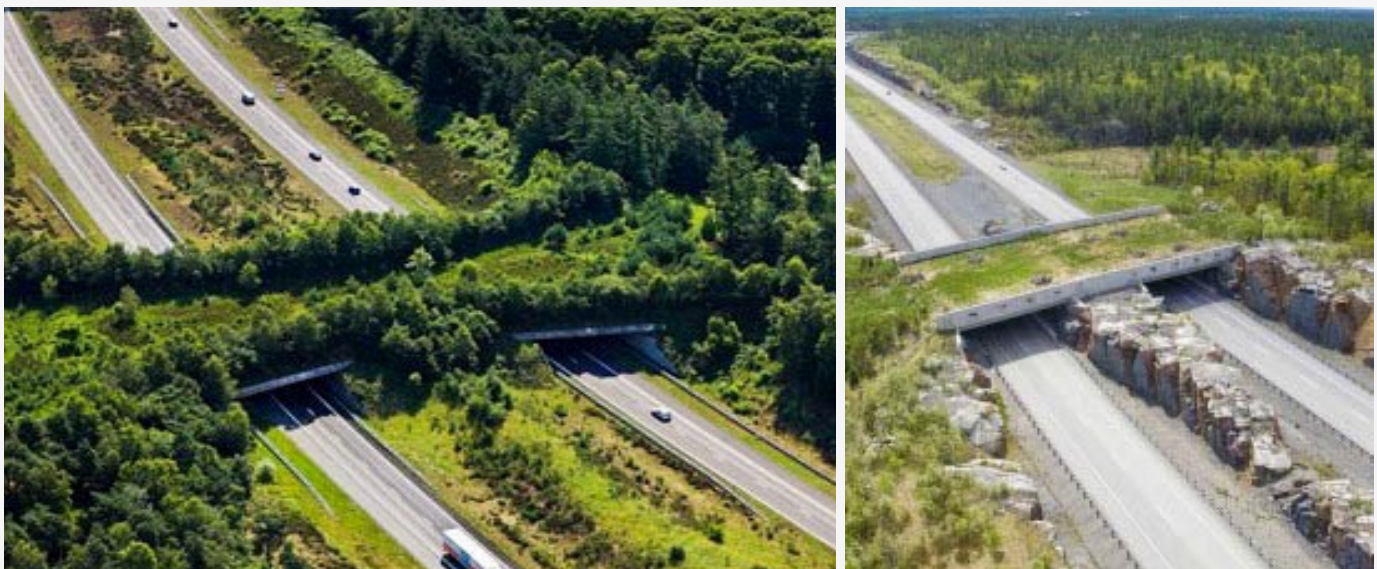
Figure 3-2 Examples of the use of vegetative screening and walls. Such measures reduce the effects of lights and noise from approaching traffic. Photo source: Siebe Swart Aerial Photography Luchtfotografie (left). Skyward Kick Productions (right).
