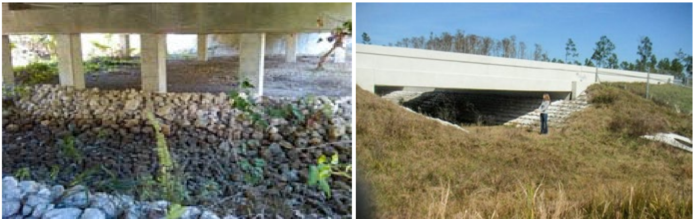
Figure 8-13 Bridges with special, seasonal-flow features (left, SR 29 in Collier County includes channel created from rip-rap; SR 40 in Volusia County includes a pipe culvert that extends through the crossing).
