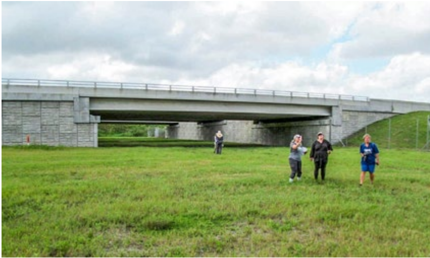
Figure 3-15 An open, single span wildlife underpass design (Wekiva Parkway).
