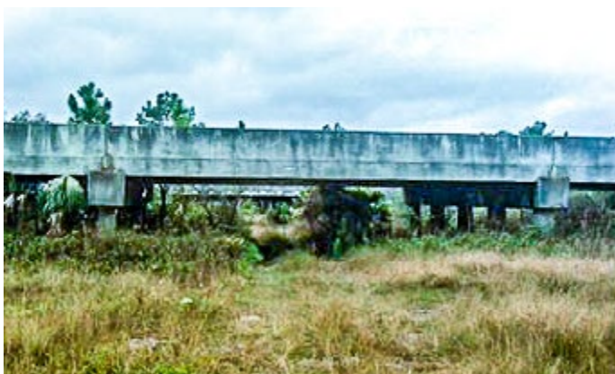
Figure 3-12 An example of a wildlife underpass typical in upland locations (I-75, Alligator Alley in Collier County).
