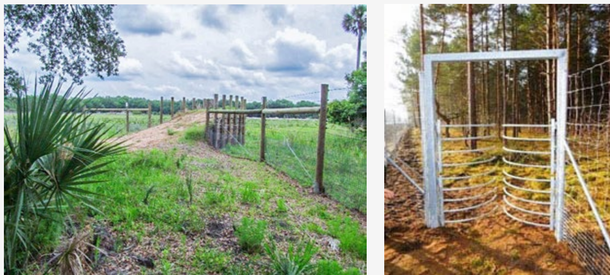
Figure 3-35 An example of a jumpout and a one-way gate; on SR 415 in Volusia County and in California, respectively.
