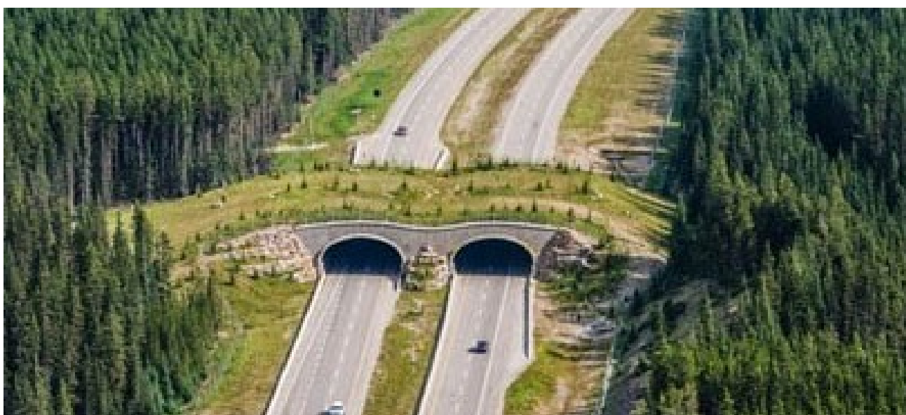
Figure 3-9 An example of an overpass of pre-cast arch sections. Photo source: Wildlife overpass in Banff National Park Photo: Parks Canada / Allie Banting / 2014.
