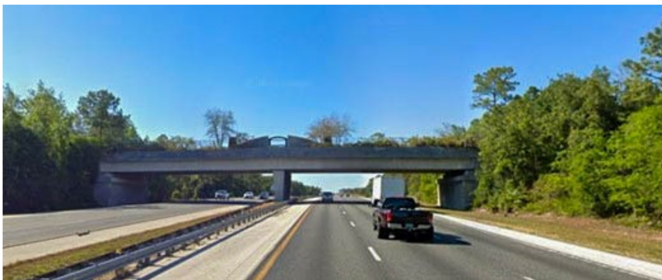
Figure 3-8 An example of an overpass with typical beams and column supports.
