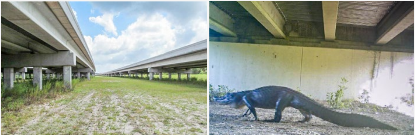
Figure 8-6 Example of underpass bridges at upland sites (left, Wekiva Parkway in Lake County; right, SR 29 in Collier County). Also see figs. 3-12 and 3-15 to 3-17.
