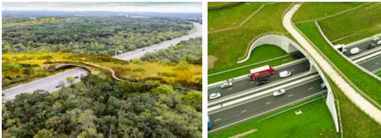
Figure 8-17 Examples of multi-purpose overpasses (Texas, upper left and Europe, center and lower right). Note the broad natural design in the upper left with an unobtrusive, imbedded trail, while in the center is a minimal design focusing centrally on the trail and nature along the margins, and finally the example in the lower right provides separate structures for trail and wildlife uses. A cost comparison would likely reveal significant differences between the three. Photo source: Phil Hardberger Park Conservancy org / STIMPSON Landscape Architects , top left. Graeme Paton , top right. ZJA Architectural Studio , right.
