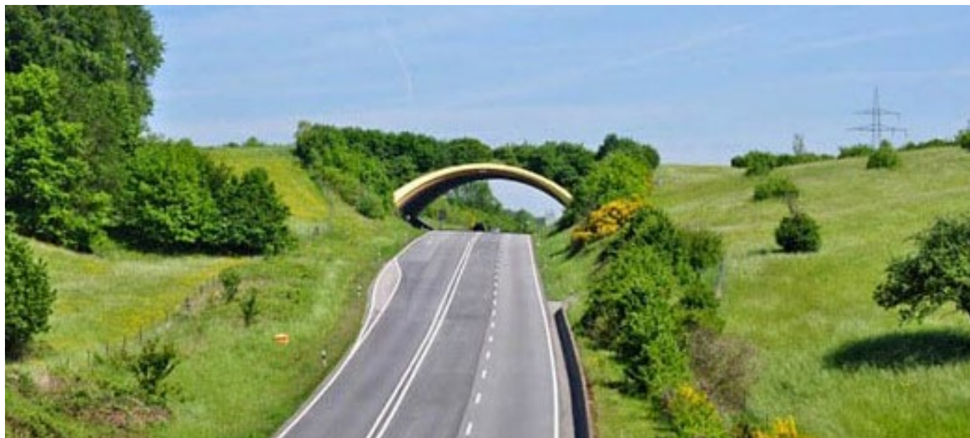
Figure 3-1 An example of a constructed overpass that takes advantage of natural topography (B38, Birkenau, Germany). This reduces the need for fill and provides minimally sloped approaches for wildlife. Photo source: Berkshire Environmental Action Team (BEAT) .
