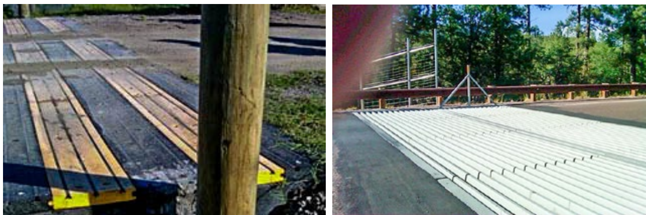
Figure 3-34 Wildlife trespass deterrents at access roads that intersect fenced road sections. An electromat device installed on an access road that intersects SR 415 in Volusia County (left), and a double-sized wildlife guard in Arizona (right).
