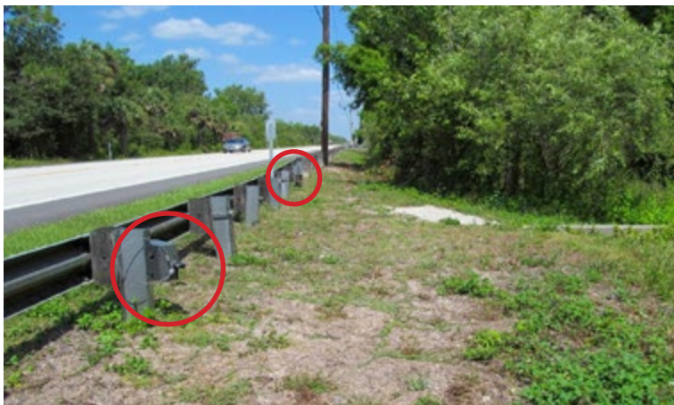
Figure 2-11 Cameras mounted on guardrail, enclosed in security boxes; on US 41 in Big Cypress National Preserve (BCNP).
