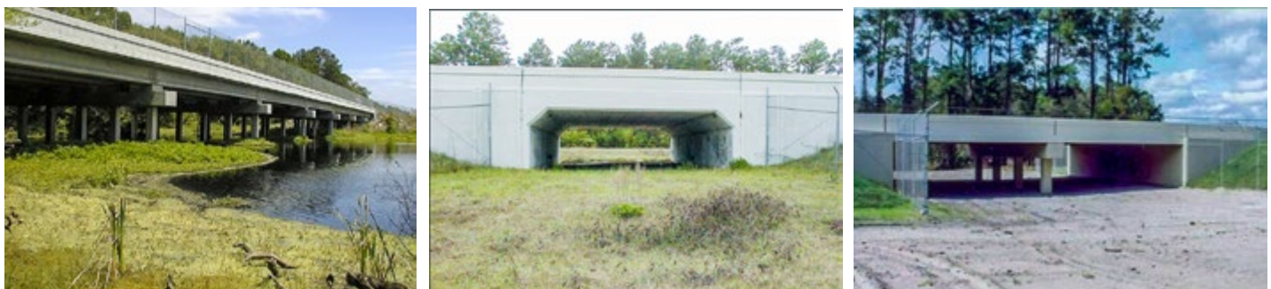
Figure 5-20 The wildlife crossings constructed on SR 46 in the 1990s and early 2000s prior to replacement by the Wekiva Parkway.
